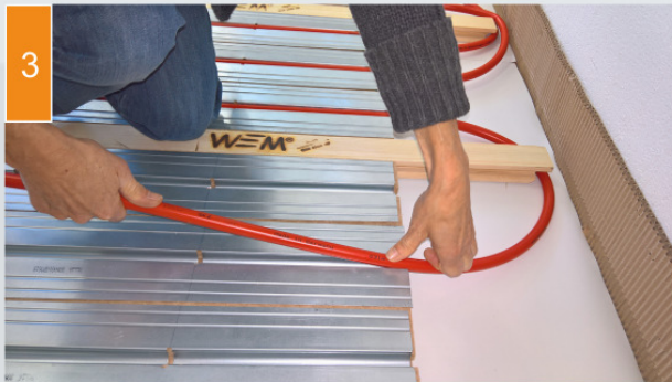
(3) The tube is inserted in the thermally conductive plates and connected to the heating manifold.
