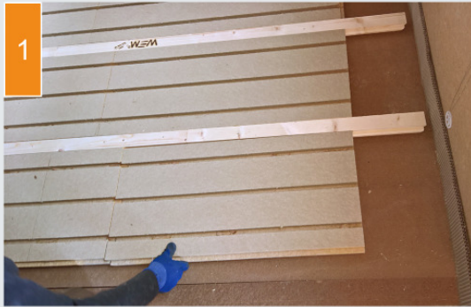
(1) The wood fibre boards and profiled frames are laid.
