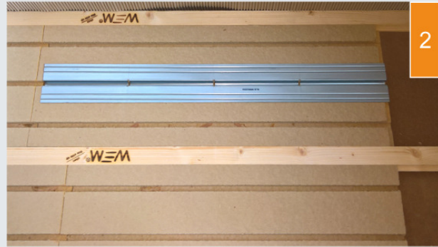
(2) Thermally conductive plates are laid in the fibre boards.
